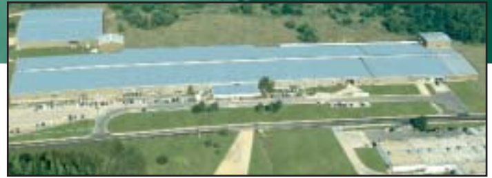
AmerCable's 400,000 sq. ft. manufacturing facility and corporate headquarters in El Dorado, Arkansas.
